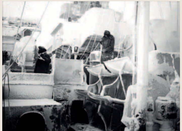
ALLIANCE: Chipping ice off the forward superstructure of HMS Manchester in Arctic waters in 1941
