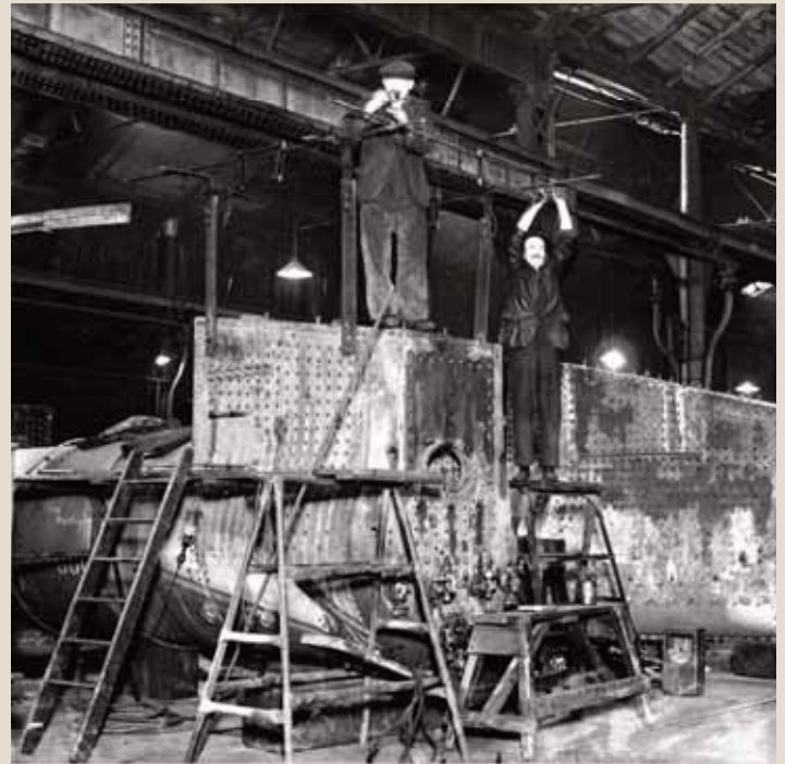
TOTAL WAR: Men working on the boiler of a steam locomotive, one of many new trains being made to keep up with the demands of the Armed Forces.
