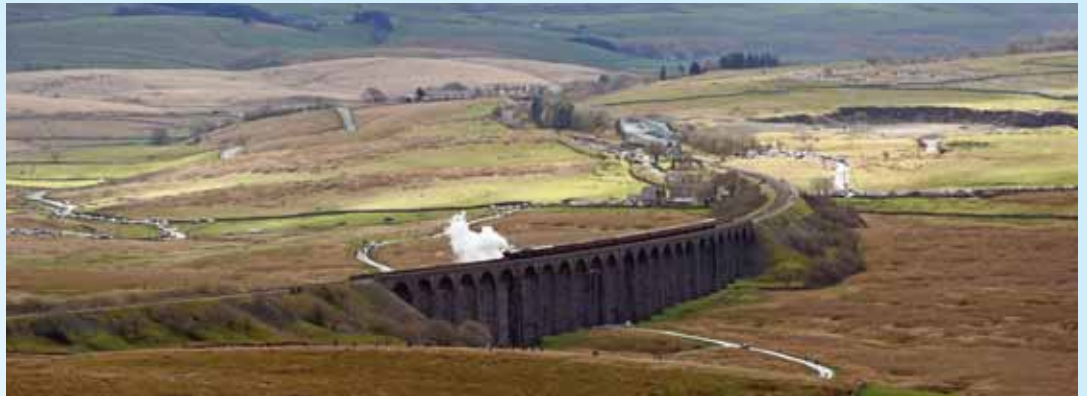
SAVED: The Flying Scotsman crosses the Ribbleshead viaduct in North Yorkshire in 2017 after the Settle-Carlisle railway line reopened following flooding.
