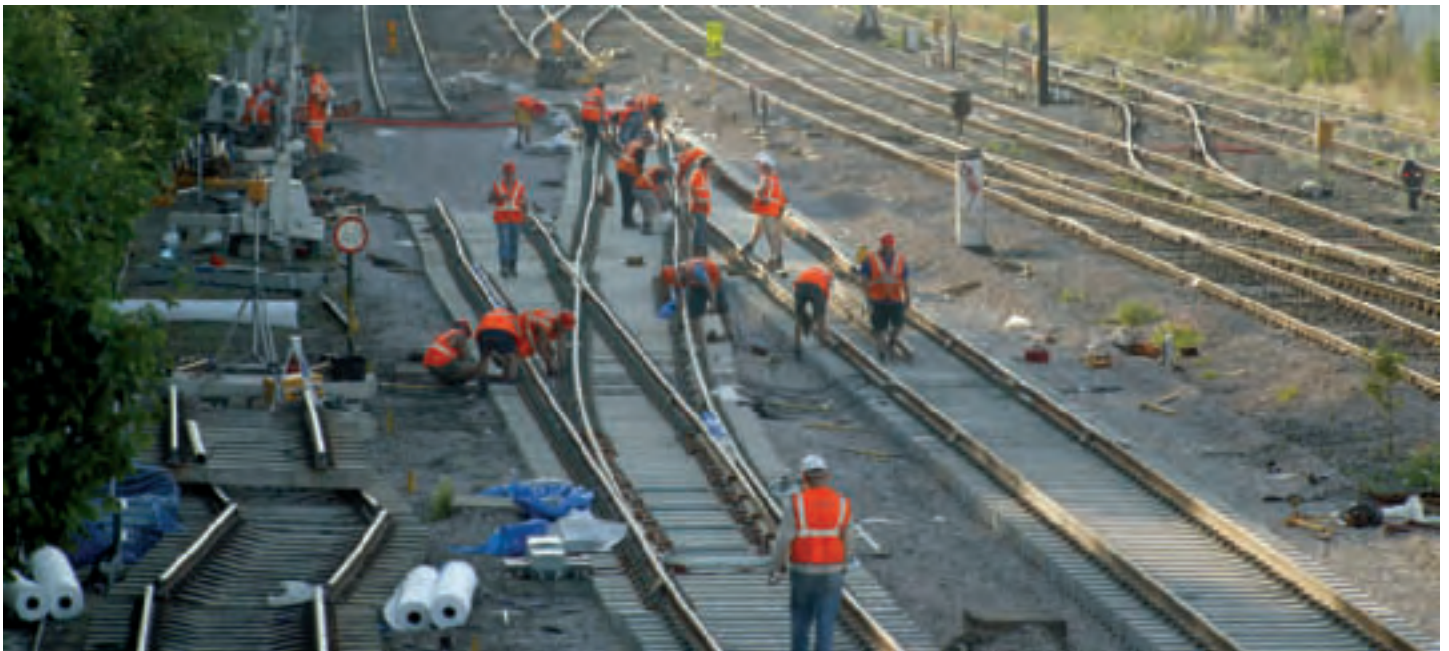
RENEWALS: Contractors Jarvis and Network Rail workers renewing worn line on the Great Western Main Line at Slough.
